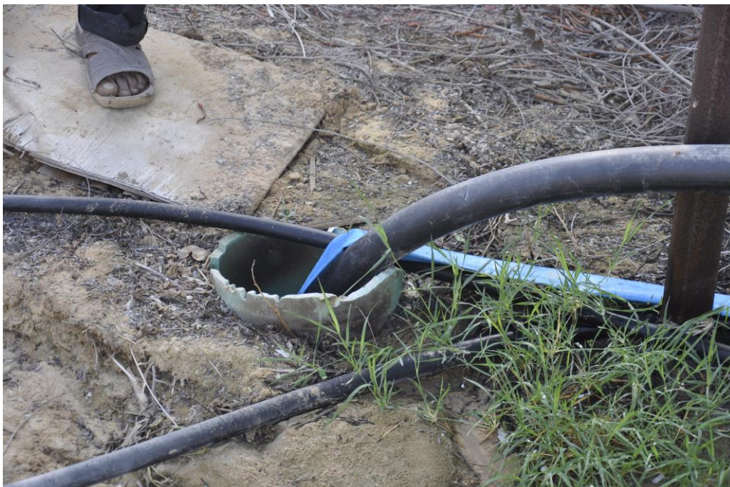
Figure 18. Brine water being deposited into an old well
