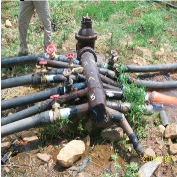
Collective well in Algeria
